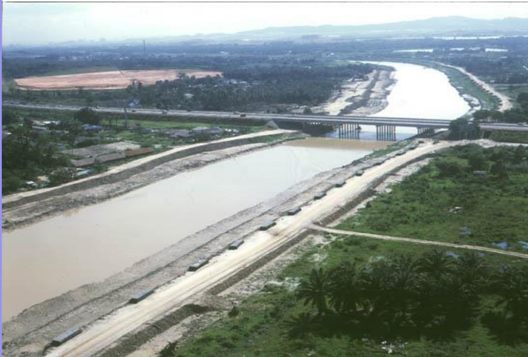
Flood Levees to protect low lying areas
